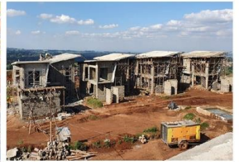
Ongoing construction of Tilisi Views
