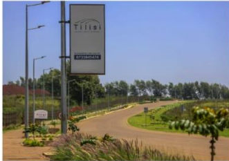
Completed Phase I infrastructure
