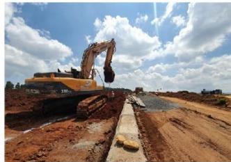
Phase II construction ongoing
